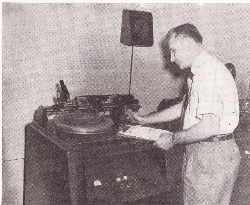
Engineer monitors the cutting of an LP with one hand on pitch control and his eyes on a cue sheet which indicates when the loud and soft passages will appear.
