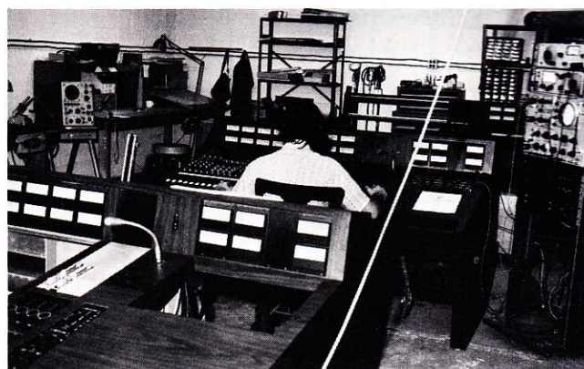
In these two photographs the console construction area is shown. Gately makes even the cabinets in his woodworking shop. With modules and components inserted, each console is given a painstaking shakedown before it goes out the door. We were told that it takes an average of seven men working one month to create a finished console.
