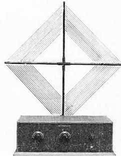
The famous Acme Reflex circuit made so easy that no technical knowledge or workmanship is necessary. You can put it together and operate it on the front porch or take it in an automobile. All of the parts for this circuit and a loop, with full sized drawings and complete instructions are included in this set, and no soldering is necessary. The only tools required for assembling are a screw driver and a pair of pliers which are contained in the kit.
